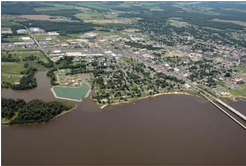
The Cambridge wastewater treatment plant, with downtown Cambridge in the background and the Choptank River Bridge on the right. Photograph by Jane Thomas, IAN Image Library ( www.ian.umces.edu/imagelibrary/ ).
