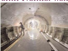
The Claremont Tunnel bypass will help our water system survive a 7.0 earthquake.
