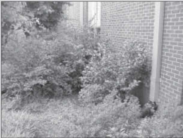
Harborage like this can lead to building invasion.
