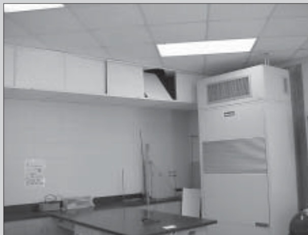
Replace missing or damaged ceiling tiles.
