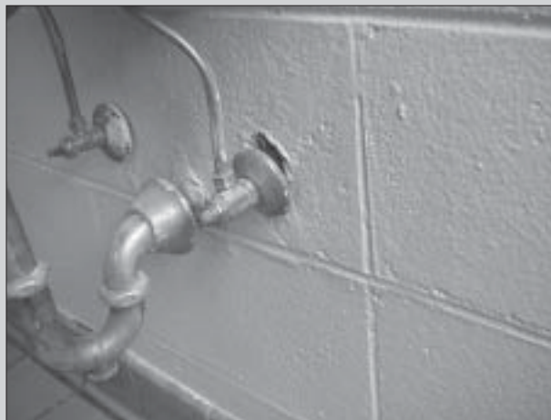
This escutcheon plate is loose. All possible pest entries should be patched, sealed or closed.
