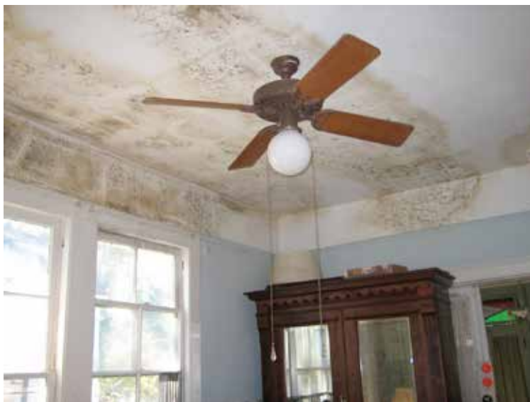
This photo of a bedroom after a roof leak during a minor storm shows significant mold damage that likely requires structural fixes, such as roof repair and replacing damaged materials. Photo by Infrogmaton.
